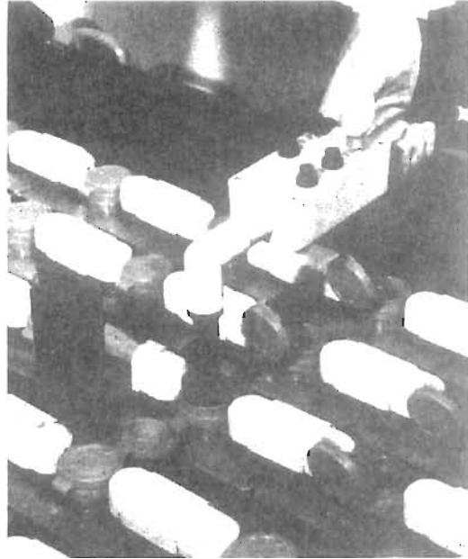
Figure 50.2 The Chloride Motive Power Battoper automatic topping-up device in use (Courtesy of Chloride Batteries)
