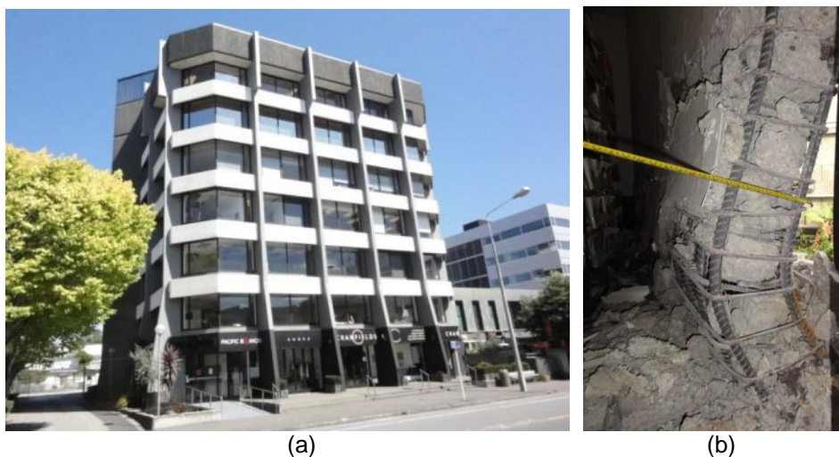
Figure 4 RC 7-storey building in Christchurch: (a) Overall view of the building; (b) wall local buckling failure (Sritharan, 2011)
